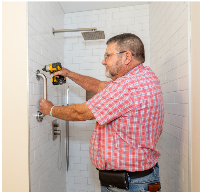
Grab bars in the bathroom to help prevent falls.
